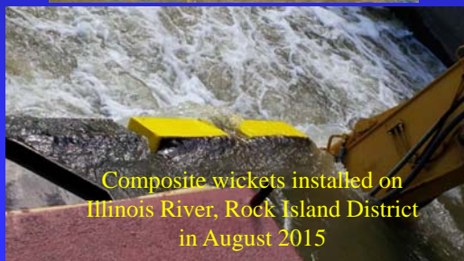
Tested to twice the working load of a timber wicket.
