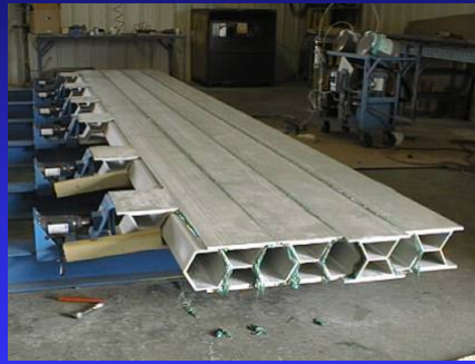
Fabrication of composite structure.
